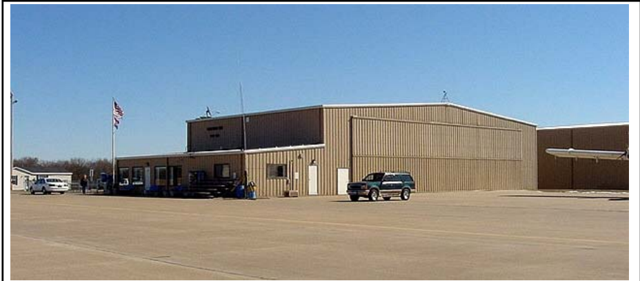
Outside view of the hangar and surrounding gathering area.
