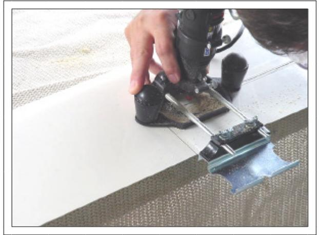
Go very slow with the cut through the end of the aileron because of the extra fiberglass, if you try to cut through this area too fast you will probably break the bit. Work the Dremel® tool down the length of the cut making sure the router base stays in good contact with the trailing edge of the aileron. Once you get to the 24" line just turn off the router and leave the tool in place until the bit stops. Flip the aileron over and repeat the cut on the bottom side.
