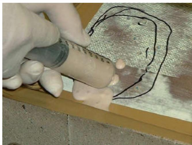
**Injecting the slurry**
