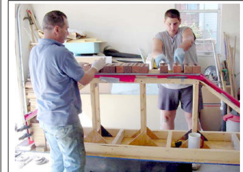
Jeff and Drew get creative with brick laying
